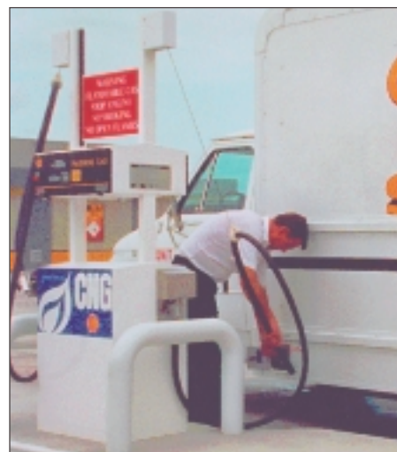
Photo 2: Conventional fuel systems are normally underground, whereas CNG systems are almost always aboveground. This brings up additional concerns for the proper management of a CNG facility. Photo courtesy of Shell Oil.
